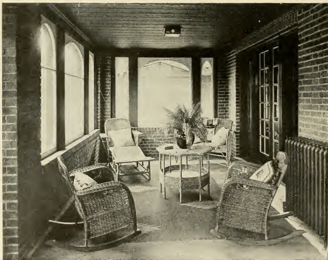
Pipes Run From Inside Radiator Warm This Porch
